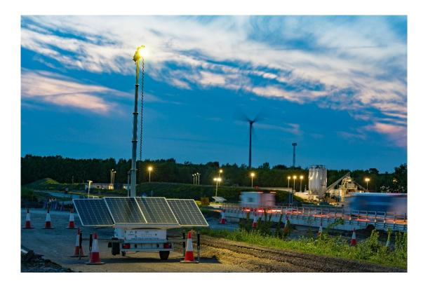
Now a total of 24 ProLights are deployed on the project in preference to diesel-powered lighting wherever possible.
